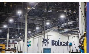
GE's Albeo LED high bay lighting fixtures have reduced annual energy use by more than 850,000 kilowatt hours (kWh) at the Bobcat facility in Wahpeton, N.D.
